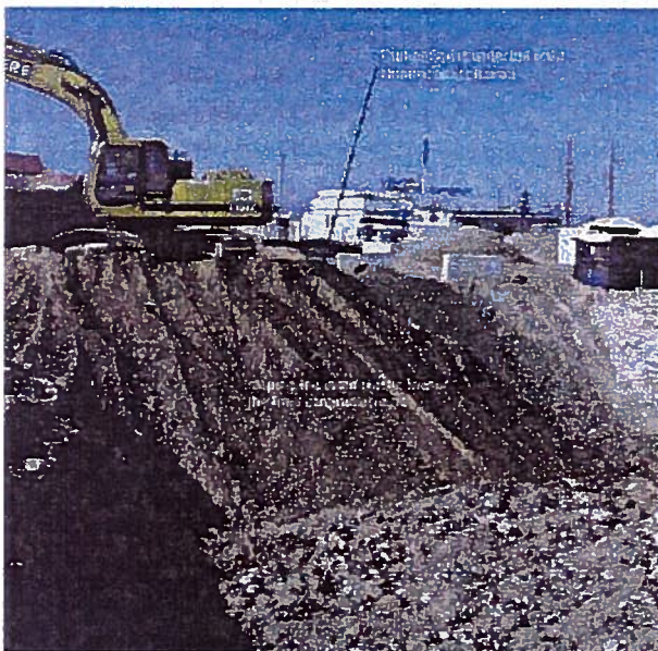
This photo shows the dark stained soil beneath the old Chromic Acid Pit. Staff of the Oversight Bureau monitor work at this Chemical Waste Landfill with Rich Kilbury dressing out in Level B to take this photo.
