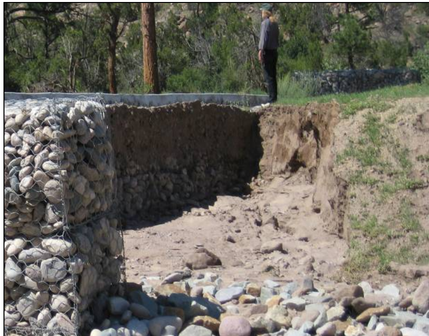
Water “Piping” caused damage in Pueblo Canyon Low-Head Weir from 8-16-10 Flood Event (upstream of weir).
