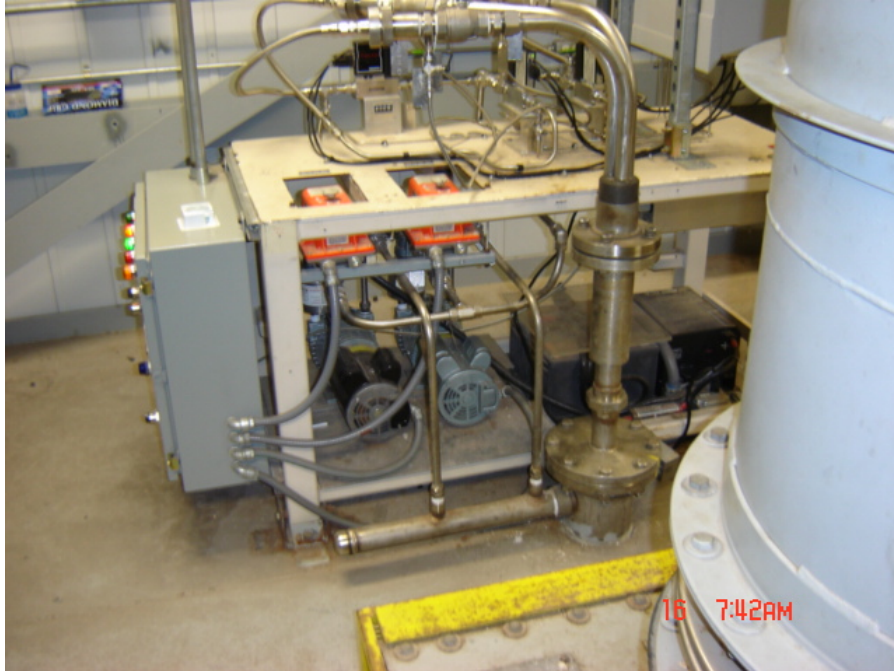
Figure WEA72-2: Inside Station A viewing one of the three filter sample sites (Skid A-2). Beneath the lower flange, a shrouded probe extends into the exhaust airshaft to focus the air stream up through the filter device above the table to collect particulates for radionuclide analysis.
