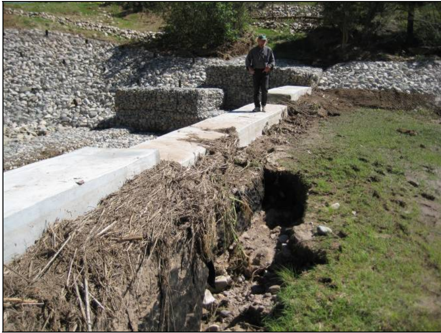
Damage to Retention Structure in Pueblo Canyon: Dave Englert assessing upstream undercut erosion damage to the Pueblo Canyon Retention Structure that occurred between 8/15 -16/2010. During the event, stormwater flowed over the top as designed, but several subsurface breaches caused substantial undercutting and break through at the structure margins.
