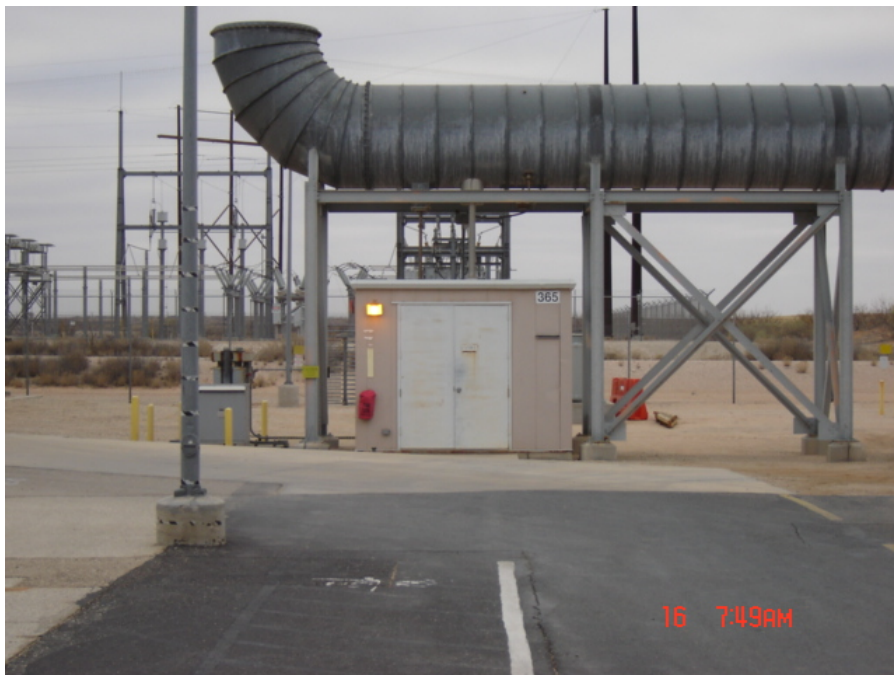
Figure WEA72-3: Station B sits below the alternate exhaust airshaft used under abnormal conditions or for tests.
