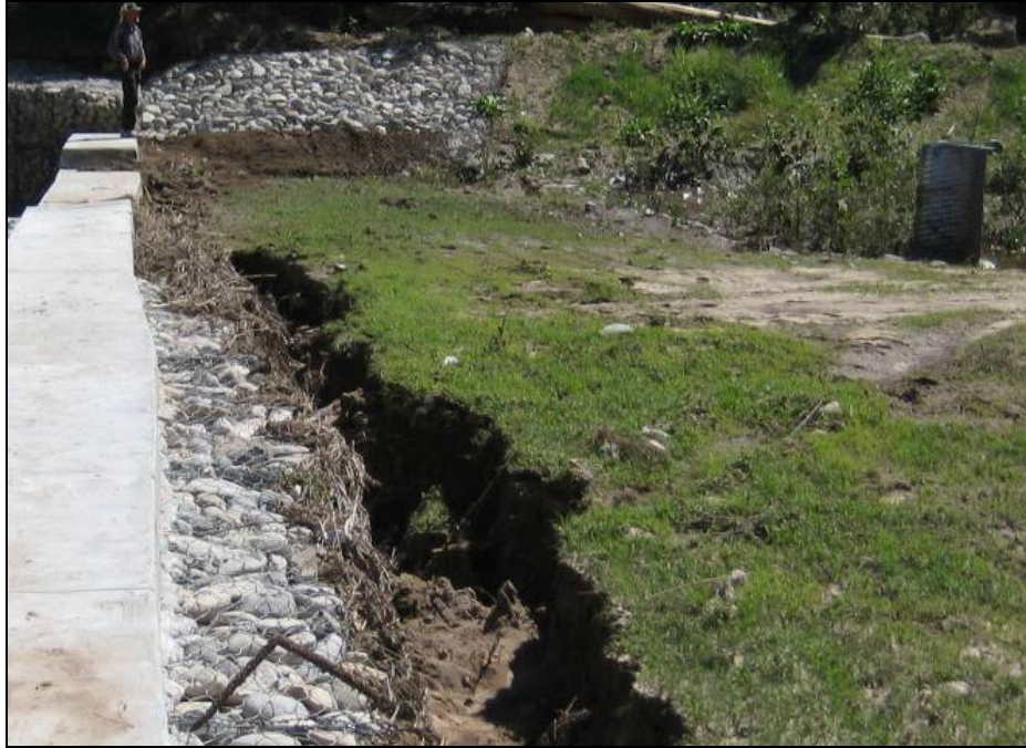
Water “Piping” caused damage in Pueblo Canyon Low-Head Weir from 8-16-10 Flood Event (downstream of weir)
