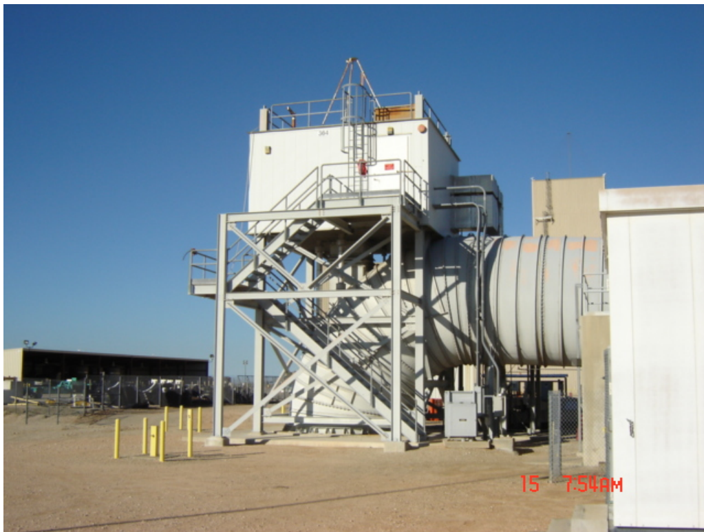
Figure WEA72-1: Monitoring Station A sits atop the 14-foot diameter main exhaust airshaft.
