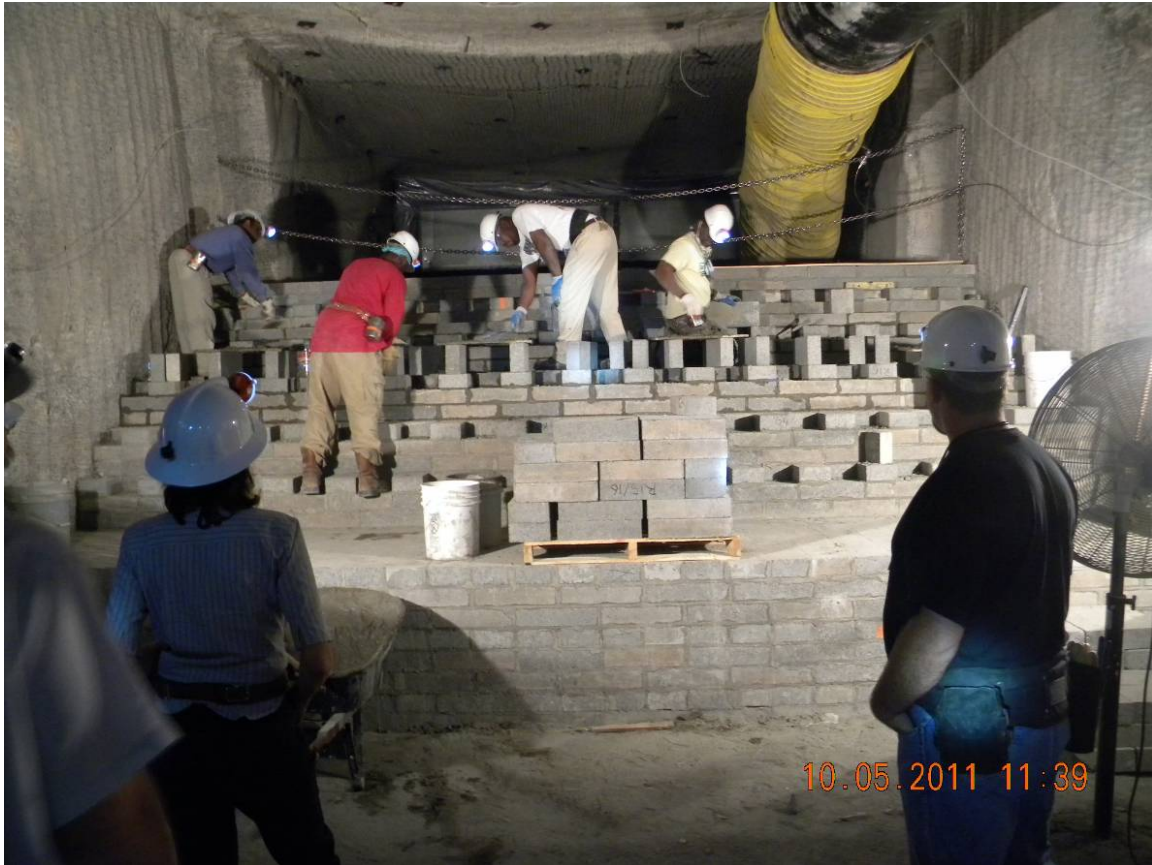
Figure WAD70-1. Contractors build the blast wall at the entrance to Panel 5.
