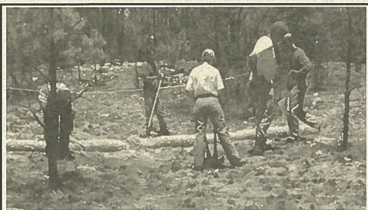
Workers install straw wattles to reduce erosion in areas affected by the Cerro Grande fire.
