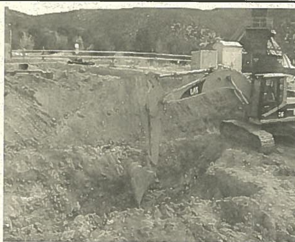
Excavation of petroleum contaminated soils below the Lurance Canyon Burn Site.
