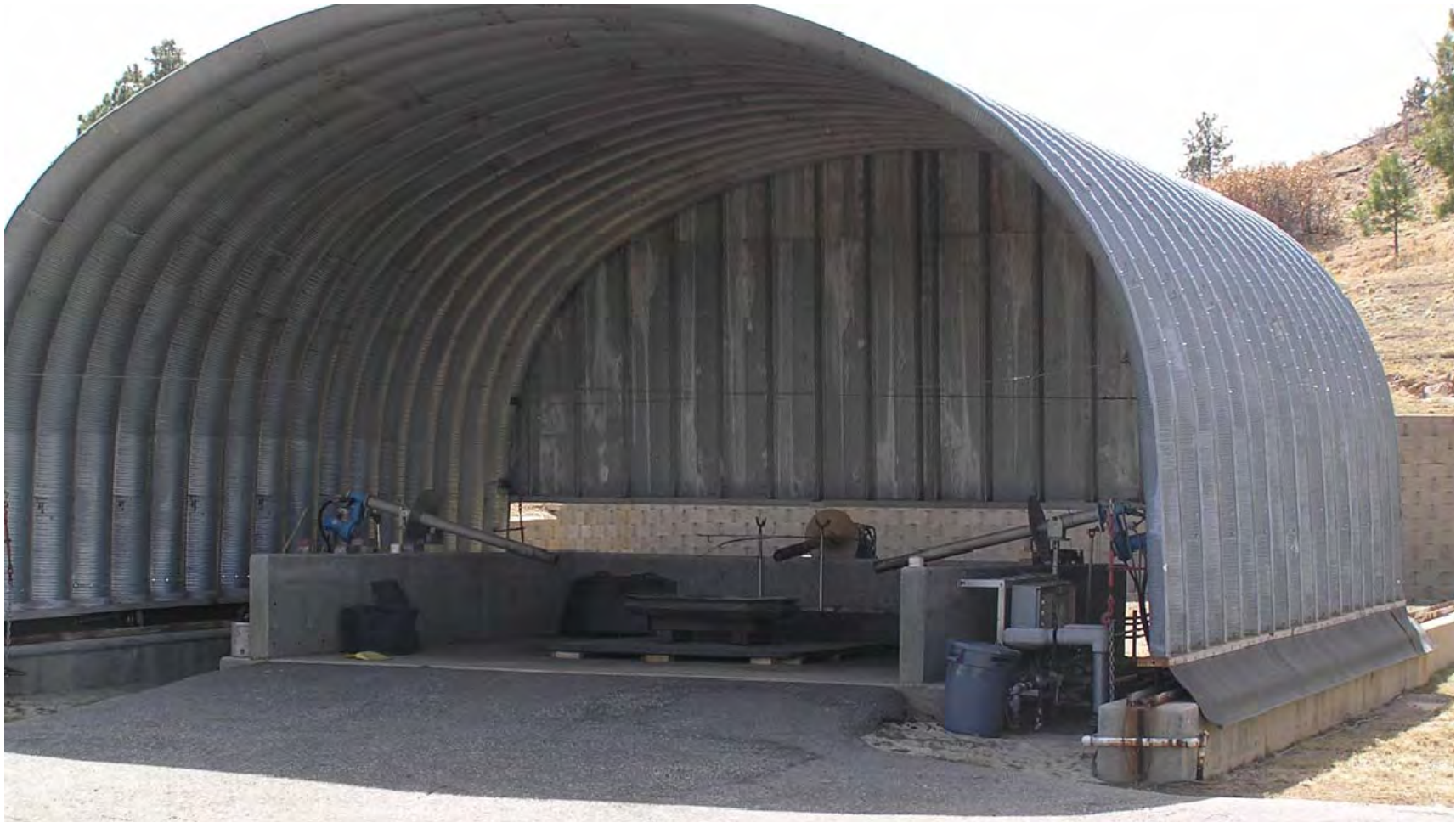
Figure 2. Current Photograph of the TA-16-388 Flash Pad (Note propane burners directed at burn area).
