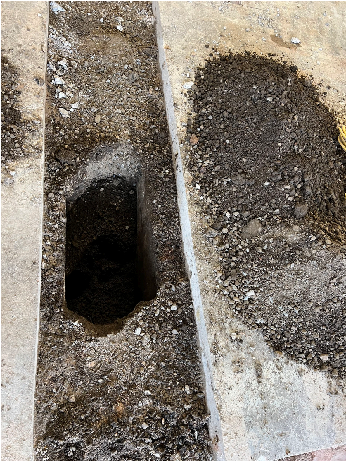
Figure 11. Photo of vault fill materials in upper 4 feet
