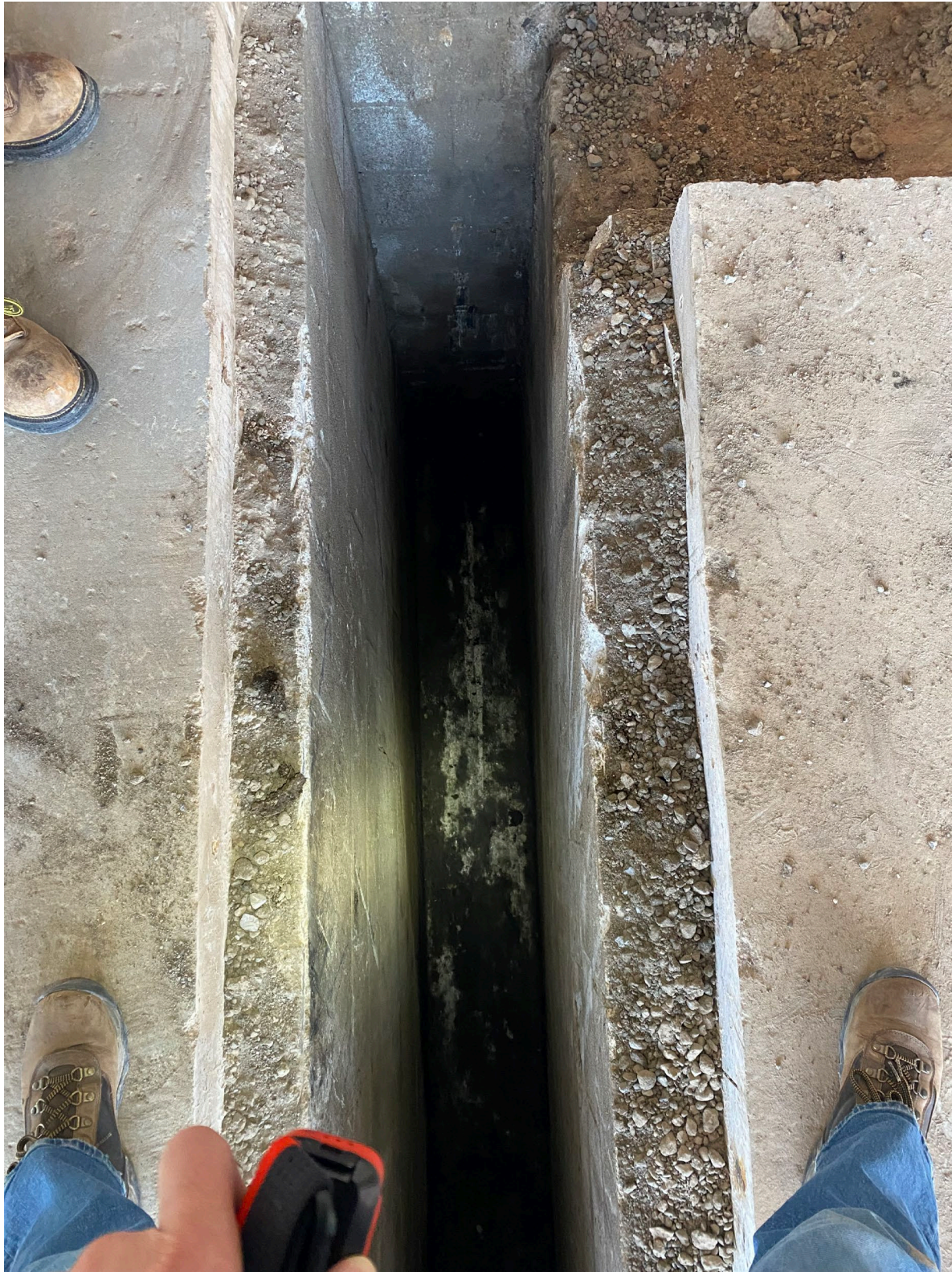
Figure 12. Photo of vault with fill materials removed
