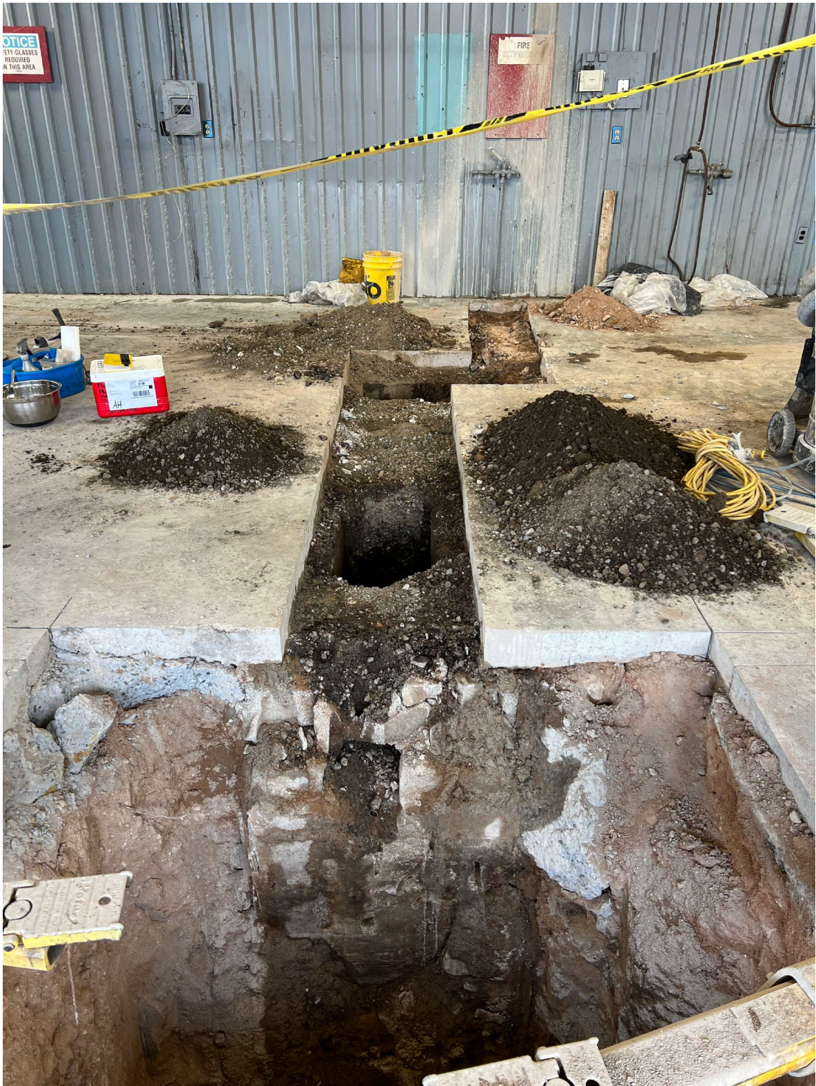
Figure 10. Photo of excavation of hydraulic lift S-2 and vault
