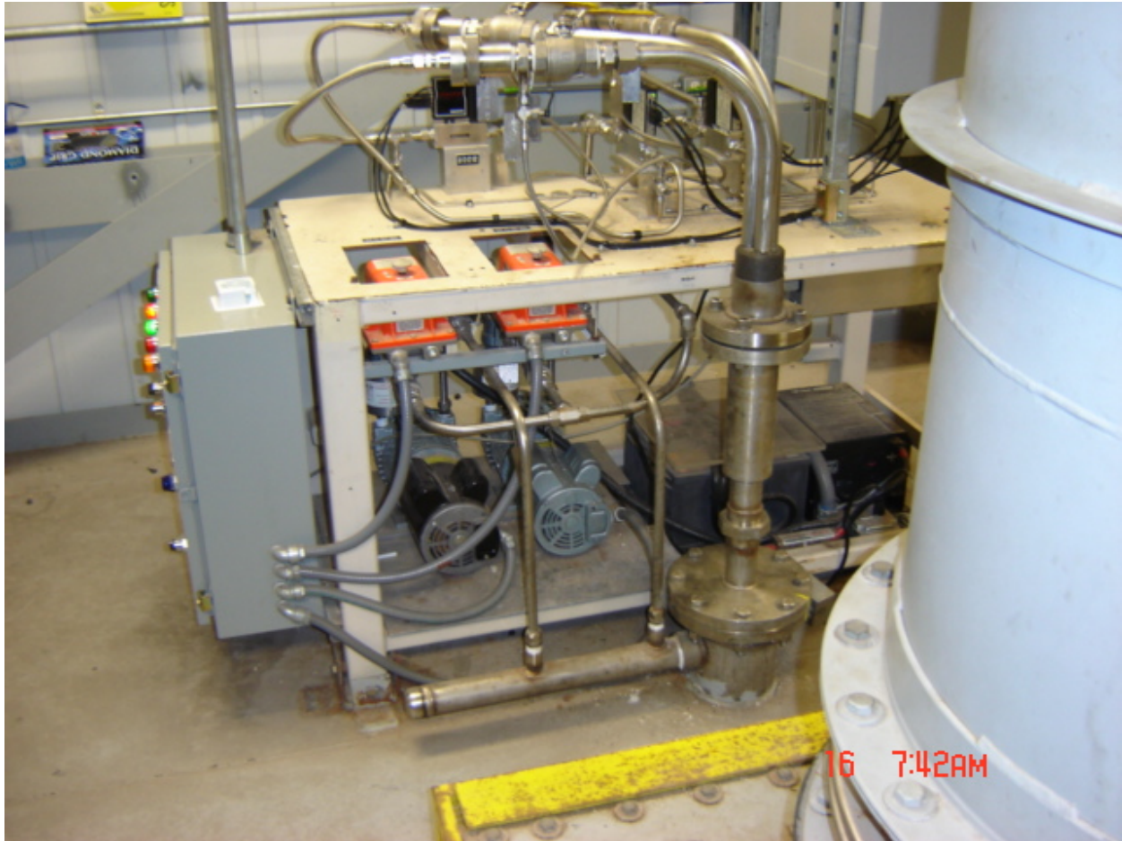
Figure WEA72-2: Interior view of one of three skids in the Station A exhaust air monitoring station. The pipe with the flange penetrating the floor carries air up through three lines to separate monitoring units housing filters above the table
