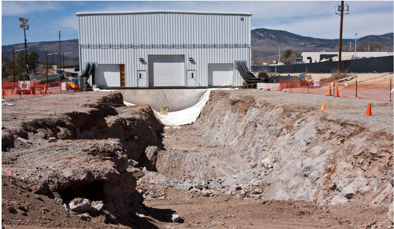
Figure LDD16-3: The trench behind moveable Enclosure 1 continues to progress with excavation. The trench will be backfilled when confirmation samples are received.
