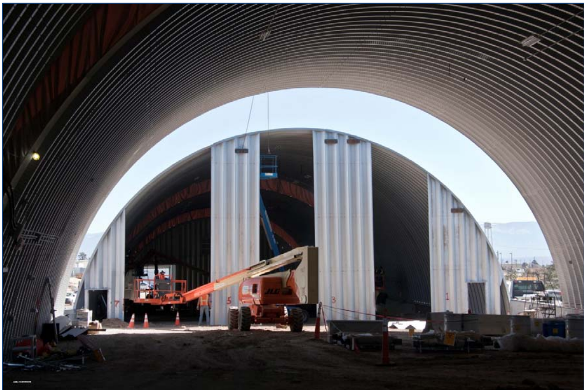
Figure LDD16-2: End panels were installed on Enclosure 5 and removed from Enclosure 3 at MDA B (TA-21).
