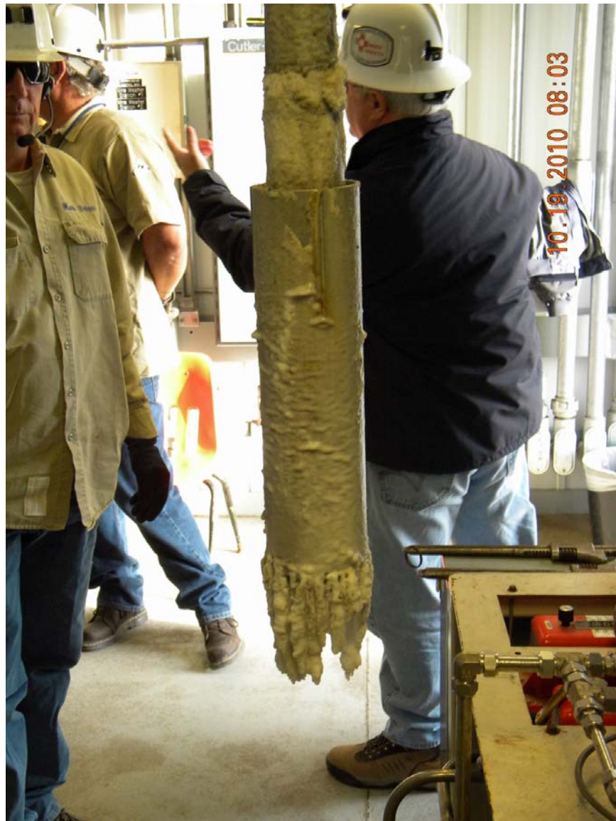
Figure WEA72-3: WTS staff removing a probe from the exhaust air shaft
