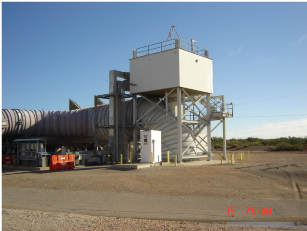
Figure WEA72-1: Exterior view of the exhaust air chamber and the Station A monitoring location at the elbow. Three probes penetrate the exhaust chamber from the monitoring station above to measure salt accumulation and to direct representative air flows to filters
