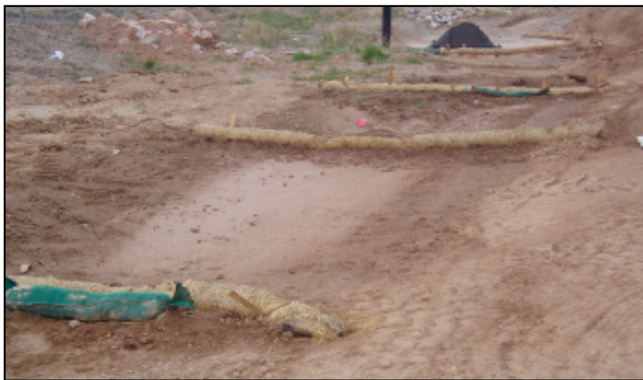
Straw wattles used at a DOE site showing deposition of sediment and flattening from “vampire” staking.
