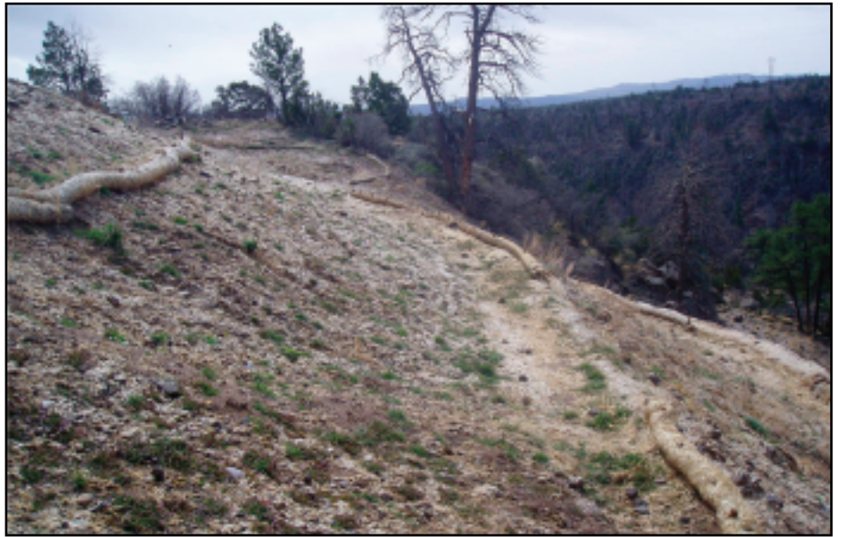
Straw wattles used at a DOE environmental remediation site (where hazardous and radioactive waste was present) showing degradation and the possibility for a contamination release.
