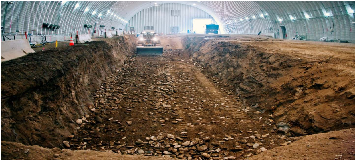
Figure LPN12-1: View of Enclosure 3 (similar to Enclosure 12) at MDA-B. Crews are filling the pit with clean fill
